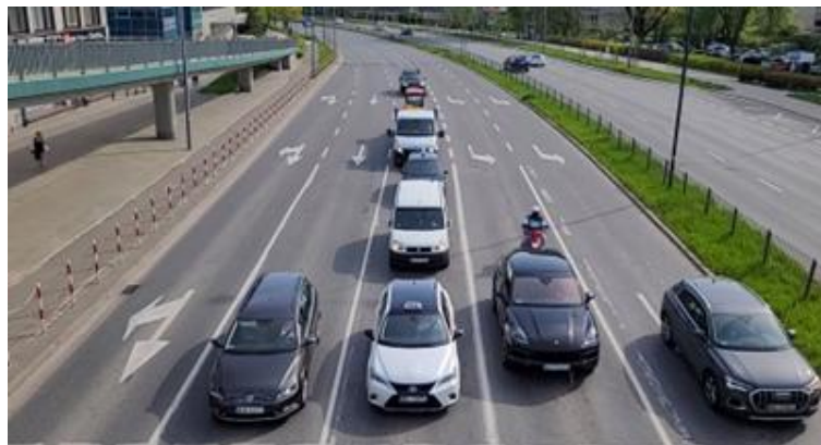
Fig. 1. View of Rzymowskiego Street, Warsaw from the perspective of the pedestrian and bicycle bridge
